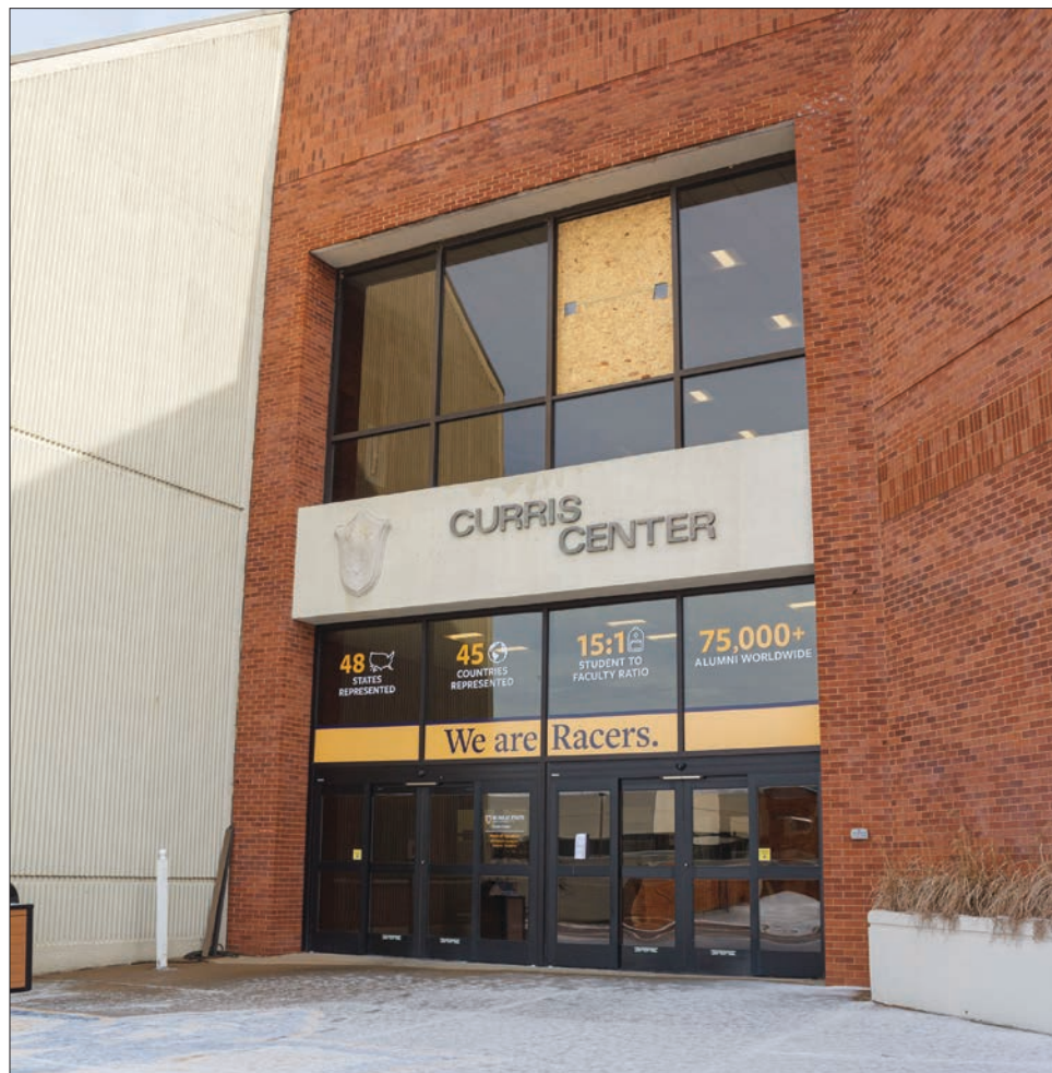
Curriss Center construction started during the Fall 2022 semester.
